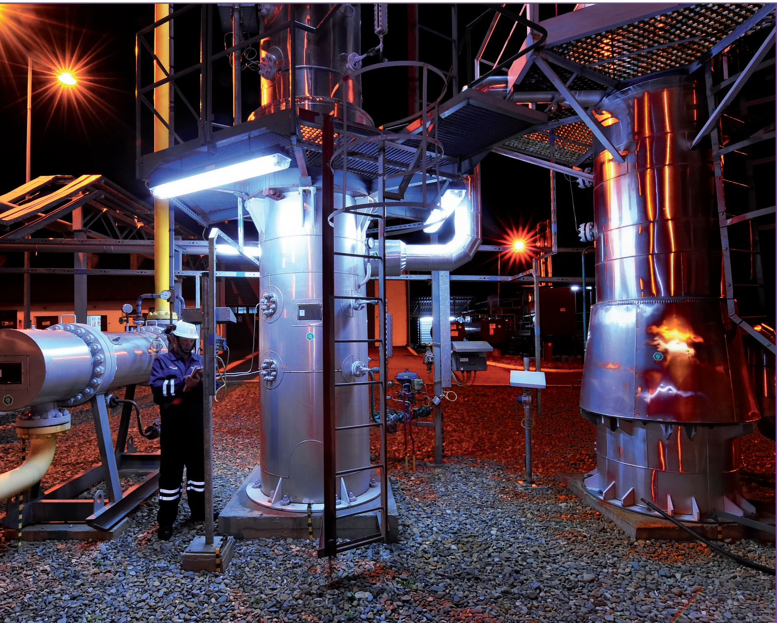
© Image courtesy of GAZ-SYSTEM - Metering station in Lasów, Poland
