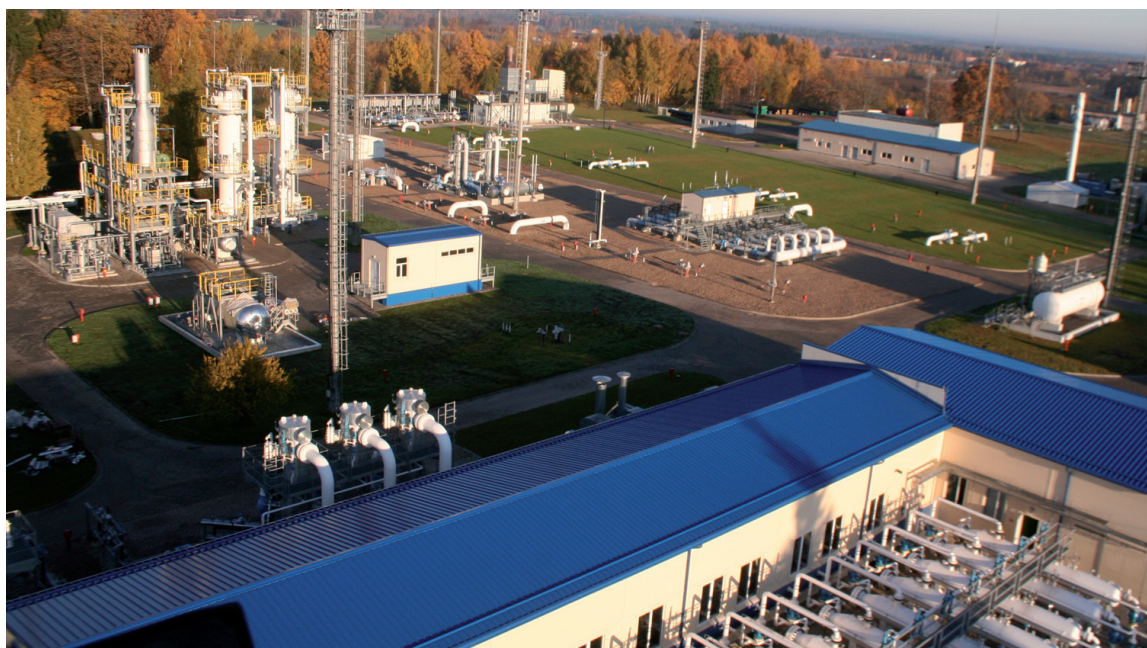
Incukalna underground storage facility
