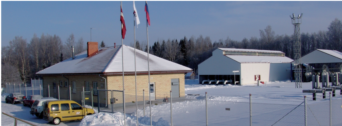
Metering station 'Korneti'
