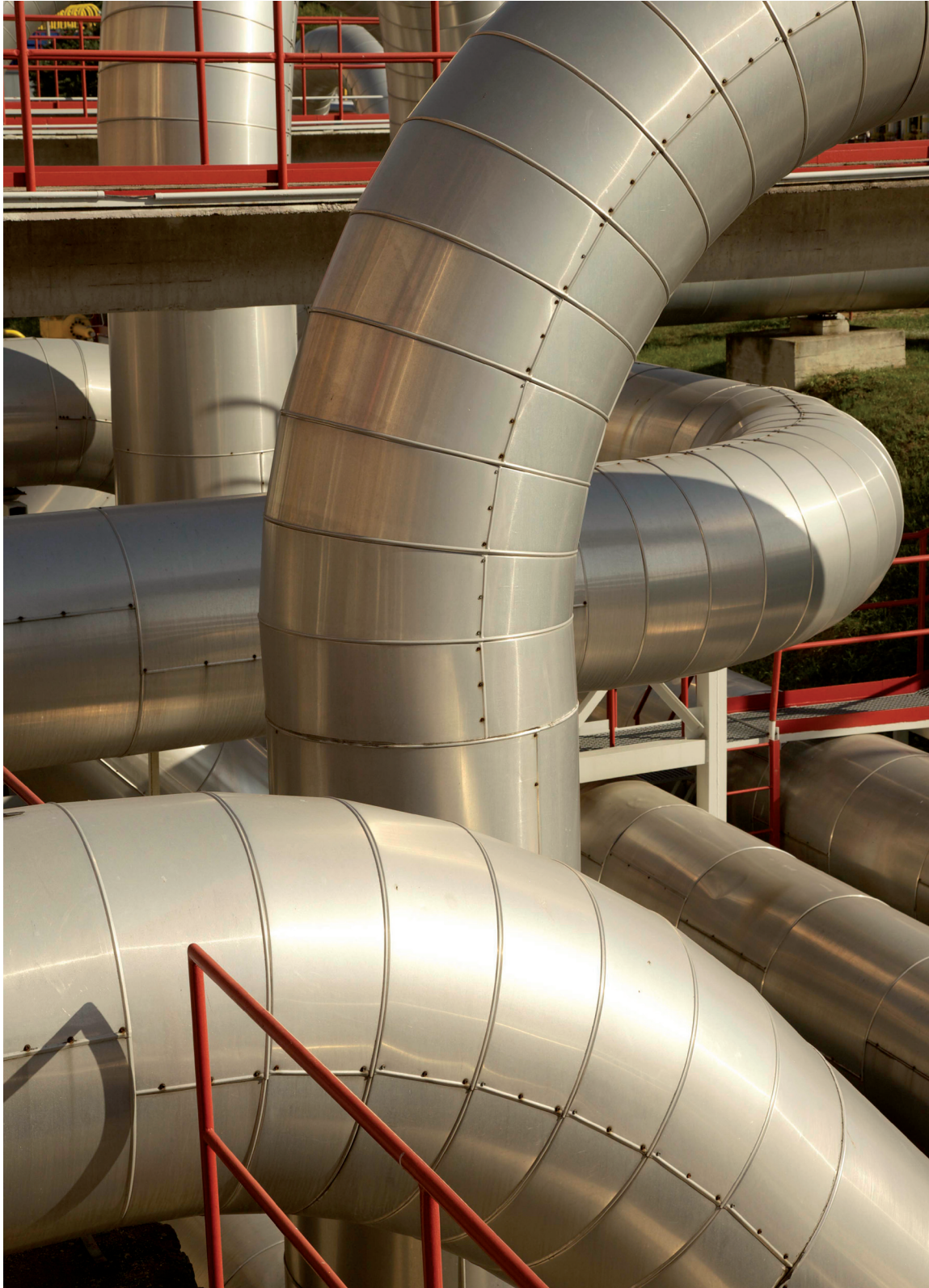
© Image courtesy of NET4GAS, s.r.o.
