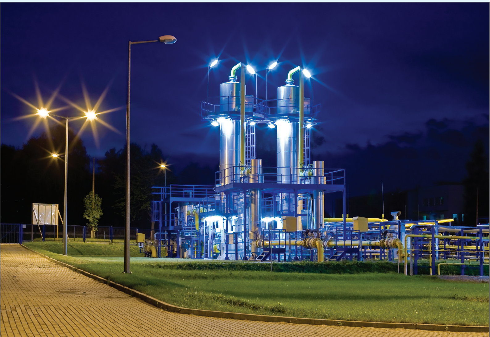
Gas dehydration station in Mackowice
