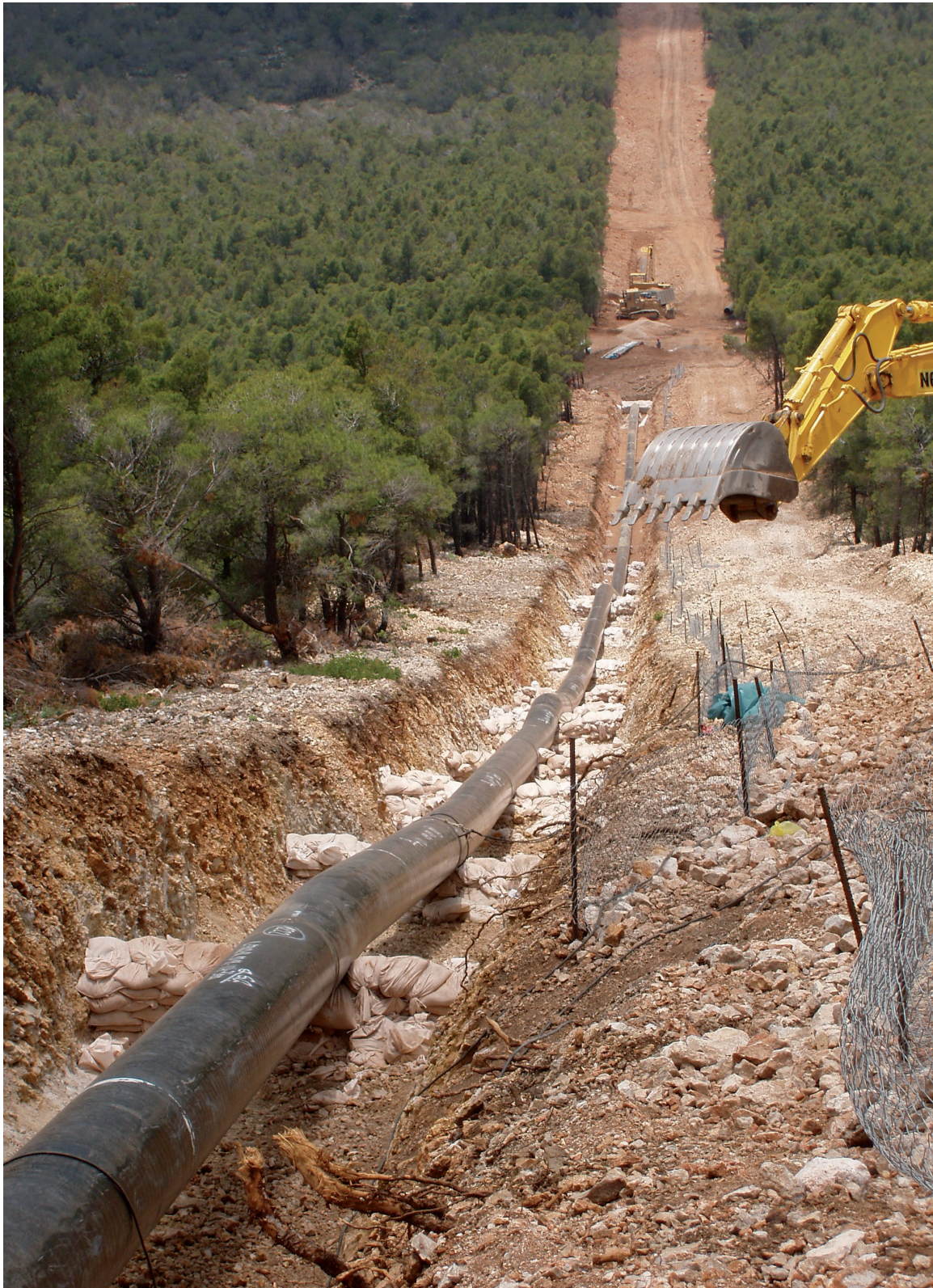
Steep slope pipeline construction in Corinth branch
