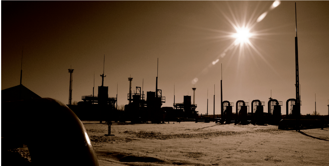
Beregdaróc compressor station
