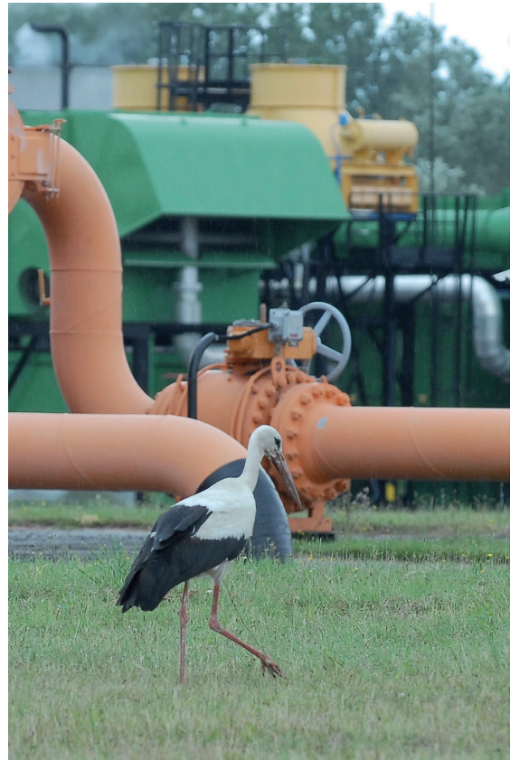
Beregdaróc compressor station
