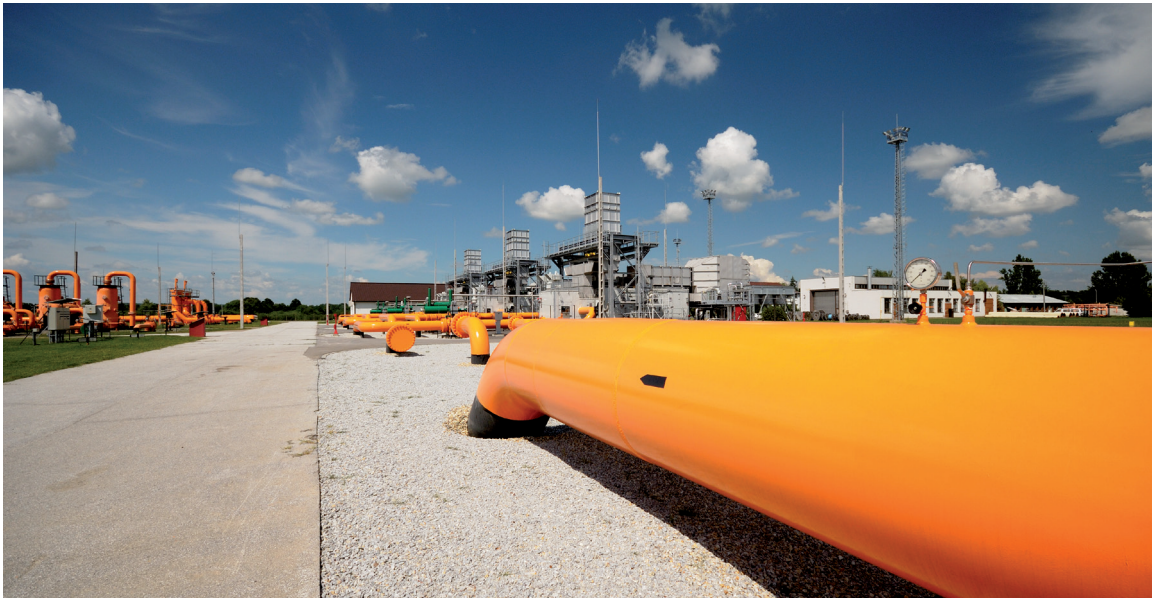
Beregdaróc compressor station
