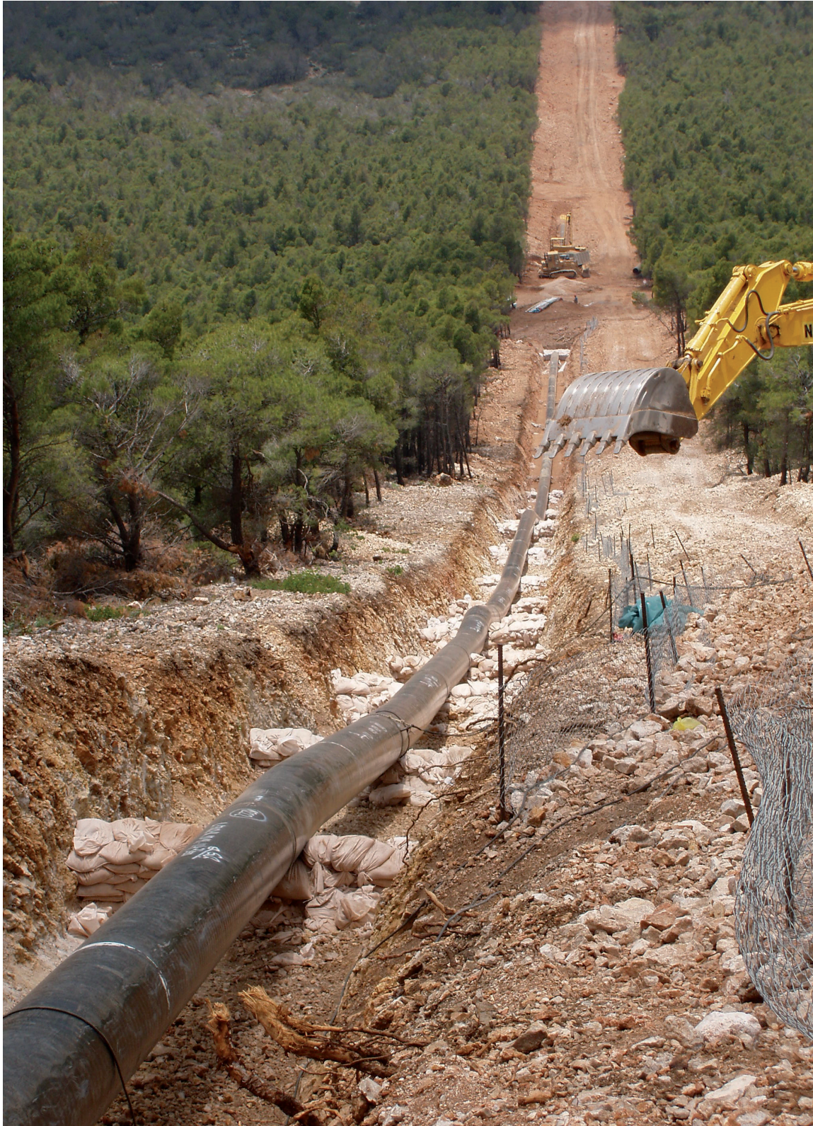
Steep slope pipeline construction in Corinth branch
