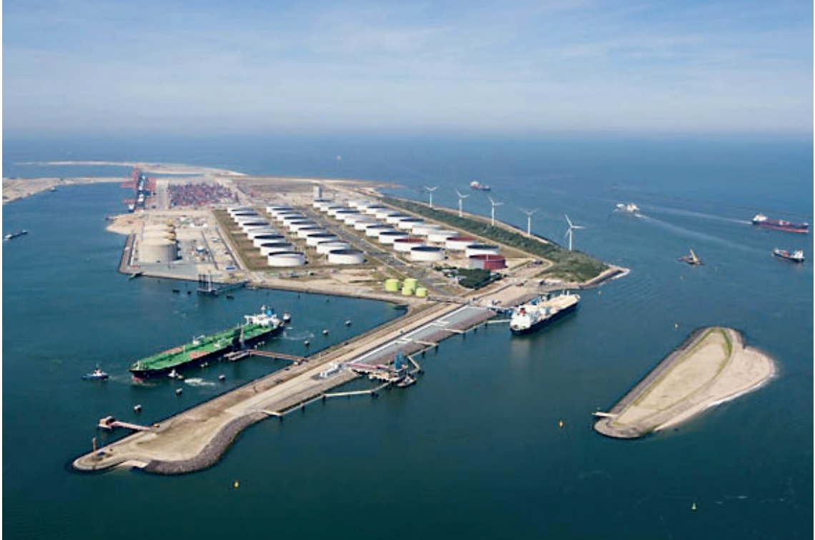
Figure 9.13: Overview of the GATE terminal in the port of Rotterdam (Source: GTS)
