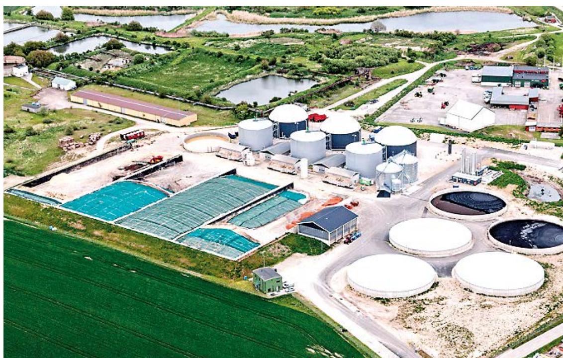
Figure 9.15: Jordberga biogas facility (Source: Swedegas)
